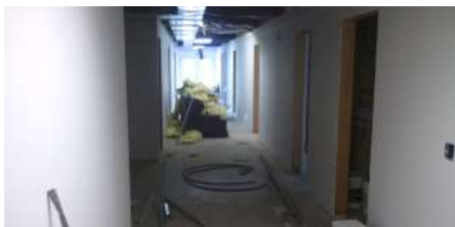
(New dormitory construction)
